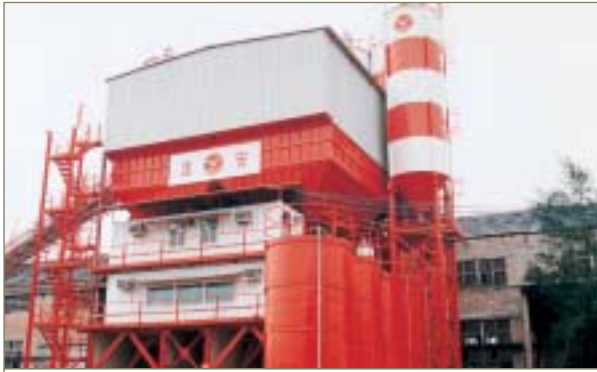
The two batching plants of Ken On in Guangzhou registered an 86% increase in output
