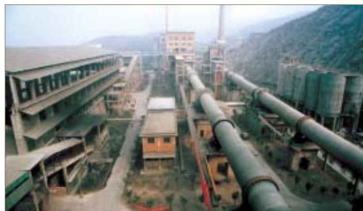
SOCAM's cement operations in Chongqing and Guizhou have gained momentum and gross annual production capacity will reach approximately 6 million tonnes by the end of the 2002-2003 financial year
