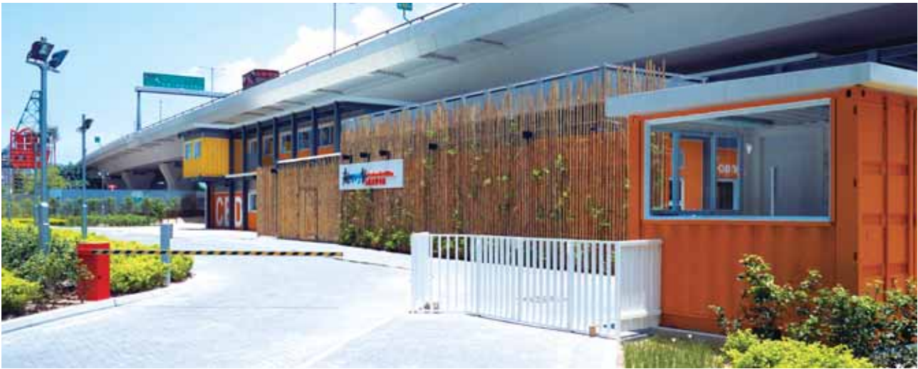
Energising Kowloon East office
